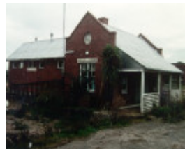
H01098 rafa barracks horse hospital demolished 1995
