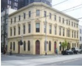
FORMER EASTERN HILL HOTEL SOHE 2008
