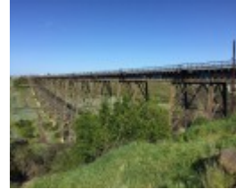
RAIL BRIDGE (ALBION VIADUCT) September 2016
