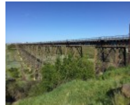
RAIL BRIDGE (ALBION VIADUCT) September 2016
