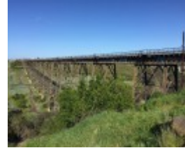
RAIL BRIDGE (ALBION VIADUCT) September 2016
