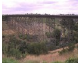
1 rail bridge albion viaduct over maribyrnong river keilor side view
