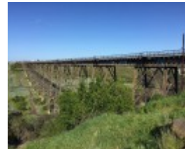
RAIL BRIDGE (ALBION VIADUCT) September 2016
