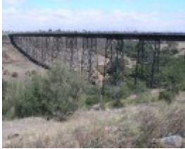
RAIL BRIDGE (ALBION VIADUCT) SOHE 2008
