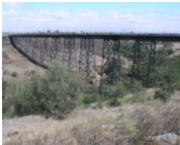
RAIL BRIDGE (ALBION VIADUCT) SOHE 2008
