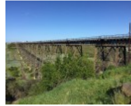
RAIL BRIDGE (ALBION VIADUCT) September 2016
