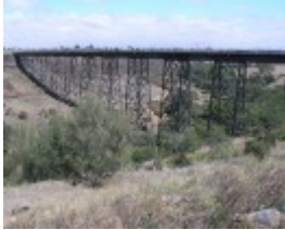
RAIL BRIDGE (ALBION VIADUCT) SOHE 2008
