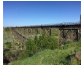
RAIL BRIDGE (ALBION VIADUCT) September 2016
