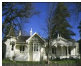
1 corio villa geelong front view
