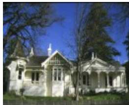
1 corio villa geelong front view
