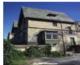
former geelong grammar school maud street geelong side view
