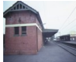
1 glenferrie railway station hawthorn station building jun1984
