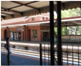
GLENFERRIE RAILWAY STATION COMPLEX SOHE 2008
