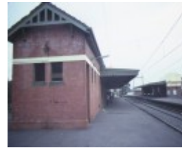
1 glenferrie railway station hawthorn station building jun1984
