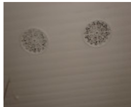
State school 2828 ventilators in ceiling KJ 26 Jul 07
