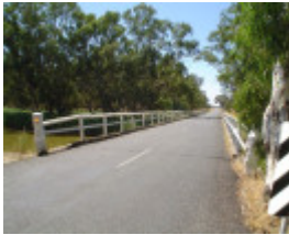
h01850 danns bridge over bet bet creek dunolly eddington road eddington across bridge she project 2004
