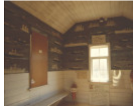
her2000 000160 1 fishermans shed interior view sw april00
