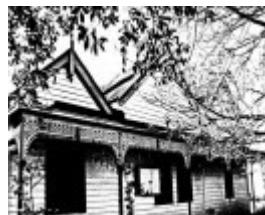
172 - Pigeon Bank Residence Kangaroo Ground 08 - Shire of Eltham Heritage Study 1992
