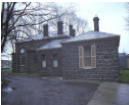
kyneton court house hutton street kyneton side elevation from rear sep1984
