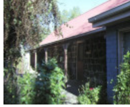
wutchach farm robert street thomastown verandah
