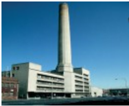
B6614 Lonsdale Street Power Station.
