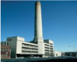
B6614 Lonsdale Street Power Station.
