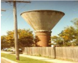
B5123 Water Tower
