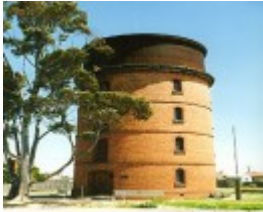
B2728 Water Tower Murtoa
