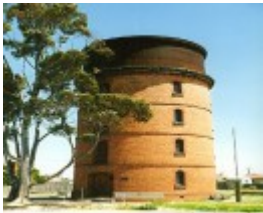
B2728 Water Tower Murtoa
