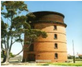
B2728 Water Tower Murtoa
