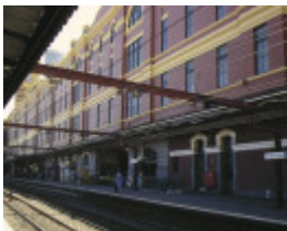
flinders street railway station complex flinders street melbourne side view
