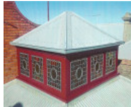
After Photograph - Reference F3907 2016
