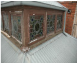
Before Photograph - Reference F3907 2014
