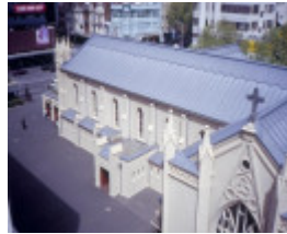
h00013 st francis catholic church lonsdale st melbourne roof she project 2003
