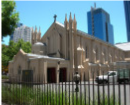
ST FRANCIS CATHOLIC CHURCH SOHE 2008
