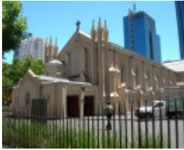
ST FRANCIS CATHOLIC CHURCH SOHE 2008
