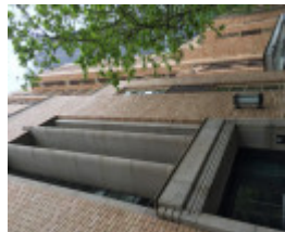
POLICE HEADQUARTERS COMPLEX Nov 2016
