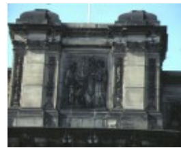
parliament house grounds works & fences spring street melbourne relief detail
