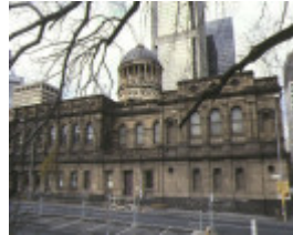
1 law courts william street melbourne side view
