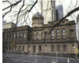
1 law courts william street melbourne side view
