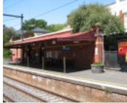
MIDDLE BRIGHTON RAILWAY STATION COMPLEX SOHE 2008
