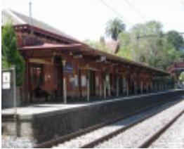
MIDDLE BRIGHTON RAILWAY STATION COMPLEX SOHE 2008
