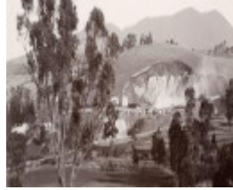
Quarry and cutting, detail (Grimwade Collection, University of Melbourne Archives).jpg
