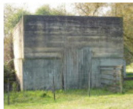
Concrete silage store from west 2017.jpg
