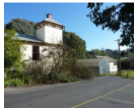
Bacon factory & timber outbuildings 2017.jpg
