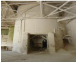
Base of No. 1 kiln 2017.jpg
