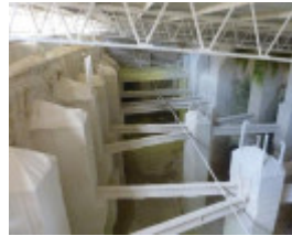
Tunnel from north 2017.jpg
