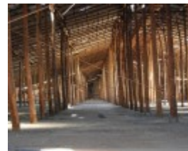
Murtoa Grain Store interior Nov 08 01
