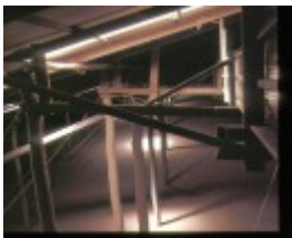
murtoa grain store wimmera hwy murtoa interior rafters
