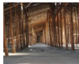
Murtoa Grain Store interior Nov 08 01
