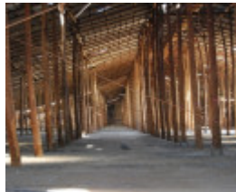
Murtoa Grain Store interior Nov 08 01
