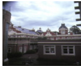
1888 building university of Melbourne parkville rear view mar1985
