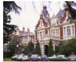
1 1888 building university of melbourne parkville front elevation
