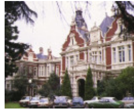
1 1888 building university of Melbourne parkville front elevation
