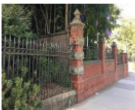
2019 Grattan Street fence.jpg
