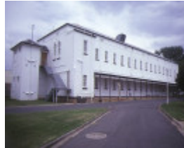
mayday hills hospital albert street beechworth rear view dec1984
