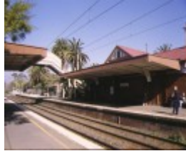
1 ripponlea railway station complex glen eira road ripponlea upside building aug1998
