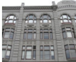
Elaborate detailing on the eastern face
