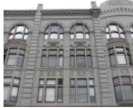
Elaborate detailing on the eastern face
