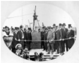
1909 - Laying of Grandstand Foundation Stone
