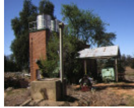
mount ophir winery stillards lane rutherglen storage tanks sep1994
