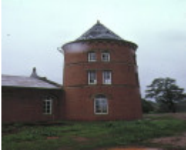
mount ophir winery stillards lane rutherglen view of tower sep1992
