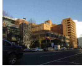
Rear and side of building (view from Nicholson Street)
