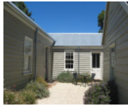
New building on left
