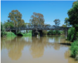
SWING BRIDGE SOHE 2008
