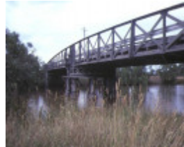
1 swing bridge over latrobe river sale side elevation feb1985
