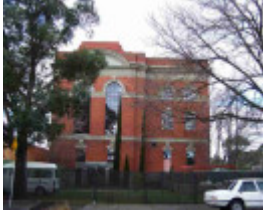
Victorian Railways DC Substation
