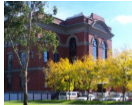
Victorian Railways DC Substation
