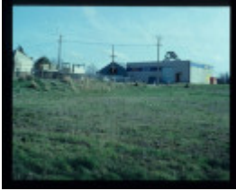
WOODEND SHELTER SHED
