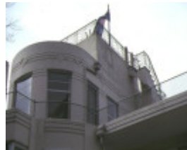
burnham beeches sherbrooke road sassafra rounded roof view
