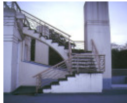
burnham beeches sherbrooke road sassafra side staircase view
