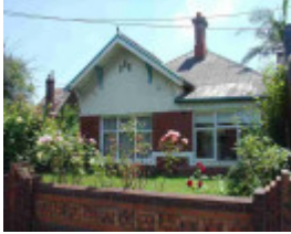
fitzroy north holden street fitzroy north holden street 195
