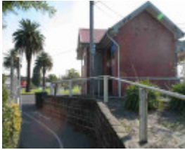
fitzroy north rushall crescent fitzroy north rushall crescent 0 off
