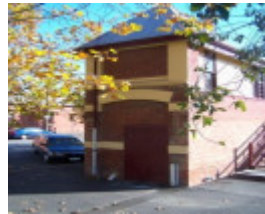
Fitzroy Cricket Club complex - Brick Gatehouse
