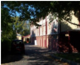
Fitzroy Cricket Club complex - Rear Grandstand
