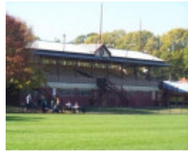
Fitzroy Cricket Club complex - Grandstand
