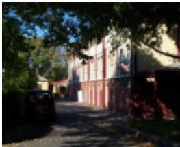
Fitzroy Cricket Club complex - Rear Grandstand
