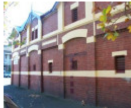
Fitzroy Cricket Club complex - Brick Gatehouse
