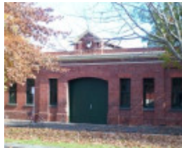
Cable Tram Engine House
