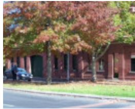
Cable Tram Engine House
