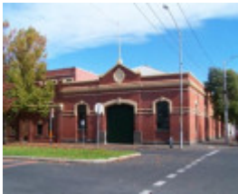
Cable Tram Engine House
