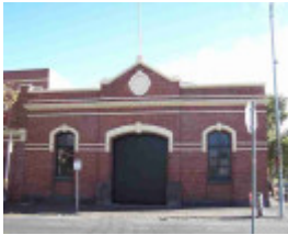
Cable Tram Engine House - 1025 Rathdowne
