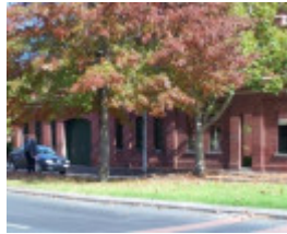
Cable Tram Engine House
