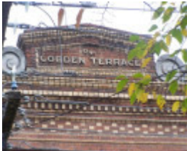
Cobden Terrace - Parapet
