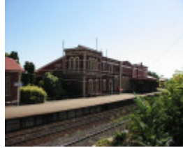
Seymour RWS Railway Building Road Side February 2002
