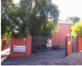
fitzroy north mckean street fitzroy north mckean street 221 unit 4
