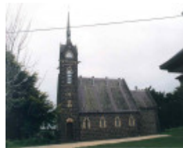
1 st andrews presbyterian church skipton side elevation 1995
