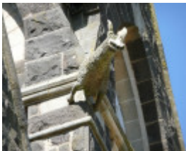
ST ANDREWS PRESBYTERIAN CHURCH SOHE 2008
