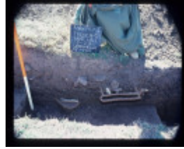
CORINELLA PENAL SETTLEMENT EXCAVATION
