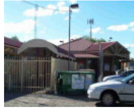
Clifton Hill Railway Station
