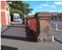
Clifton Hill Railway Station
