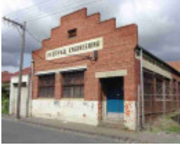
fitzroy argyle street fitzroy argyle street 160
