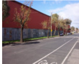
Former Coal Shed.JPG
