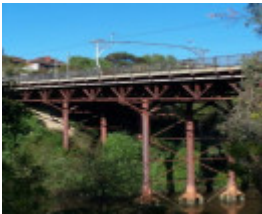
Victoria Street Bridge
