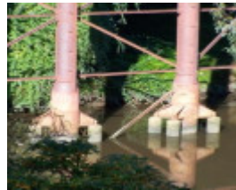
Victoria Street Bridge
