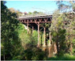
Victoria Street Bridge
