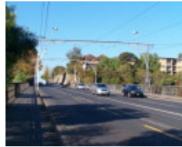
Victoria Street Bridge
