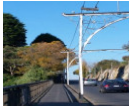
Victoria Street Bridge
