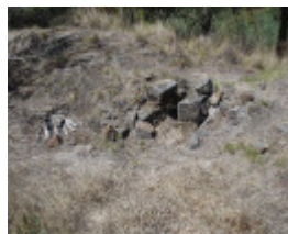
Thomas Mill - site visit 3/2/15
